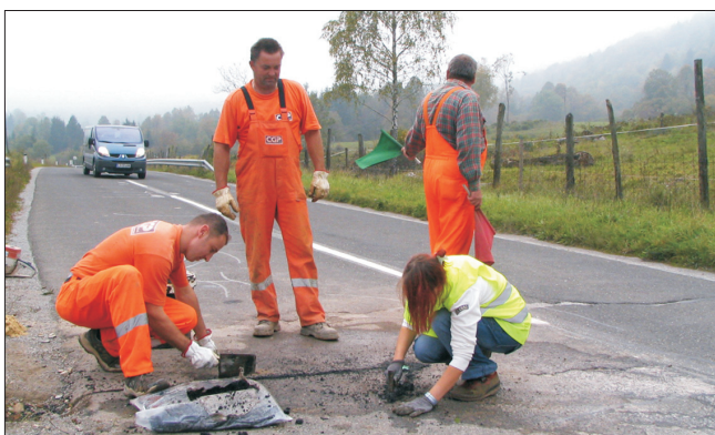
Installation of an embedded road sensor (Foto: CGS Labs d.o.o.)
